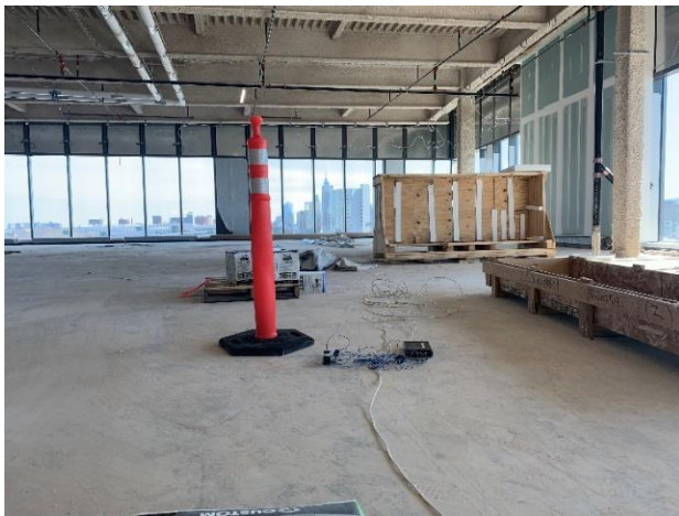
Figure 6. Existing conditions during testing
